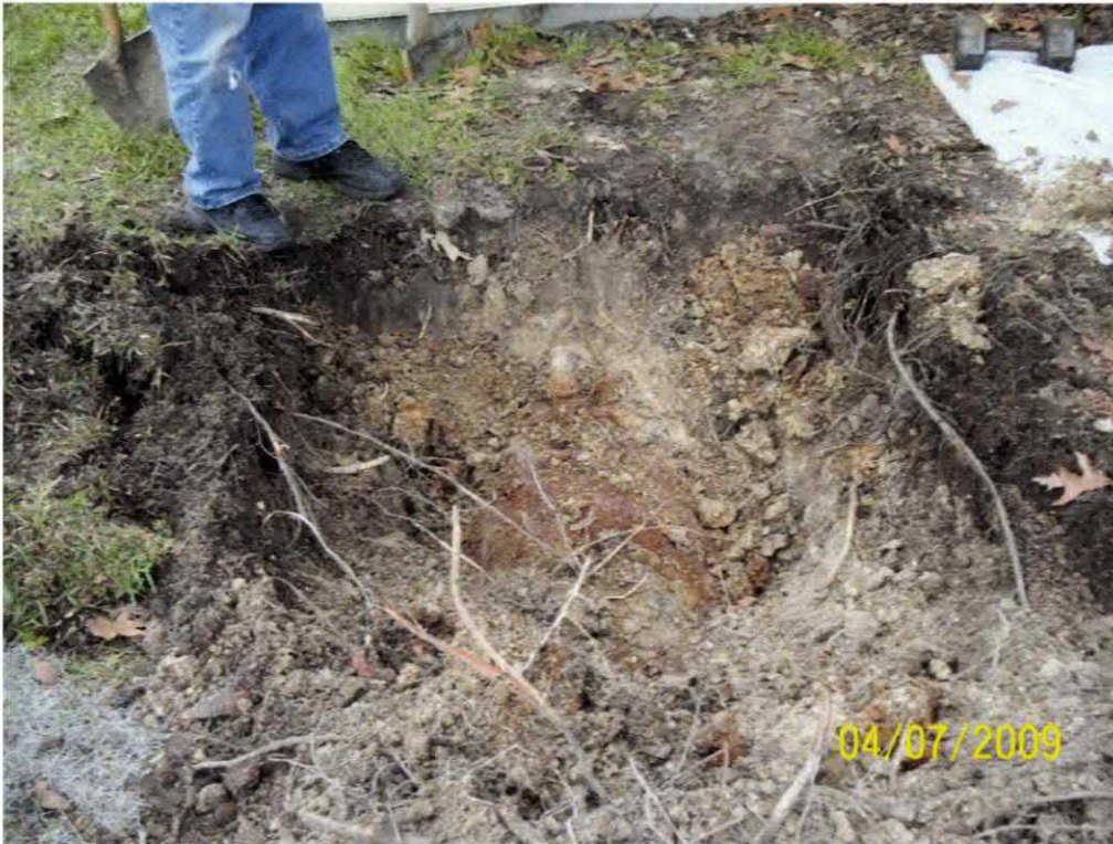
Picture 1: Top of UST 255Beech-1 exposed during removal.
