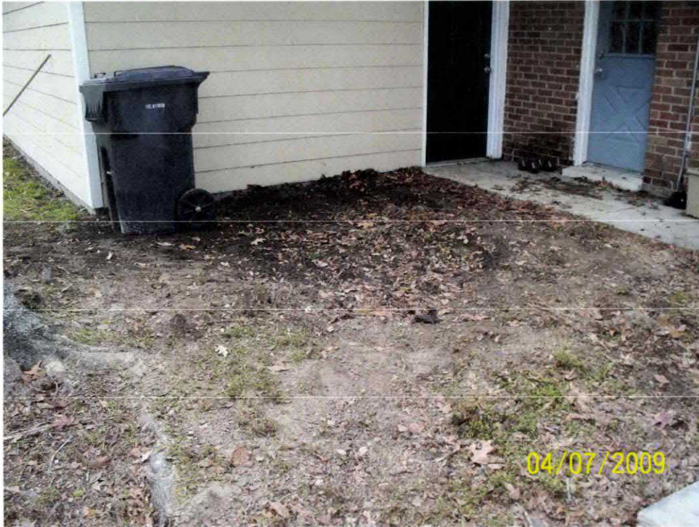
Picture 3: 255 Beech Street site at completion. Tanks were located behind garage.
